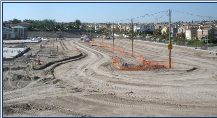
Grading for front parking lot. Tower of Building 100 is in left background.
