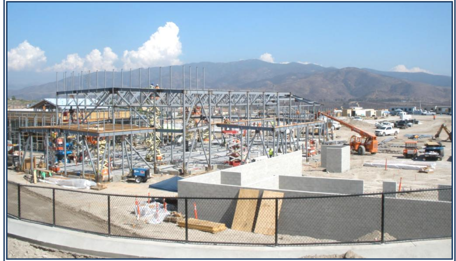
Structural steel being installed for Building 200.
