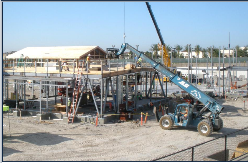
↑ Wood framing of roof on Building 100.
