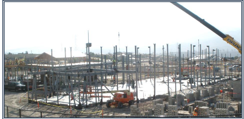
↑ Structural steel being installed for Building 200.
