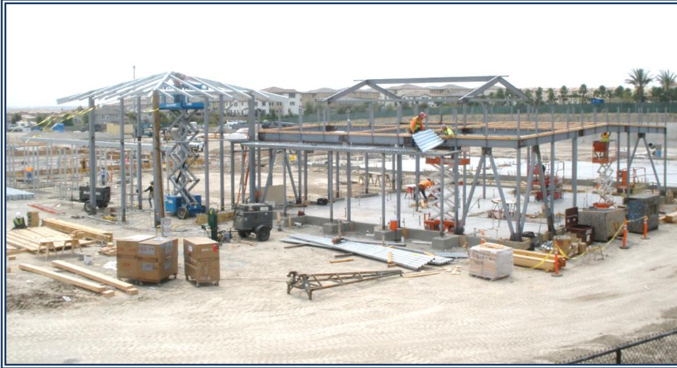
Building 100: Welding rafters on tower, framing roof, and laying metal deck.
