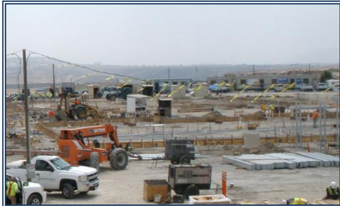
Building 300: Edge forms and under slab electrical and plumbing in progress.
