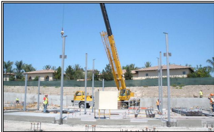
Structural steel being installed on Building 100.
