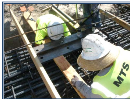
Anchor bolts being installed for Building 300.
